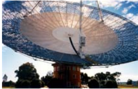
Radio dish D = 64 meters Wavelength = 20 cm = 0.02 m
