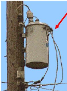
This is a typical step-down transformers used to bring the line voltage down from 5000 V to 240 V before it gets to your home
